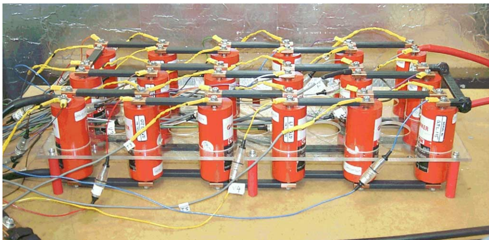
Fig. 4. 36 V battery of twin tab spiral wound cells on test.
